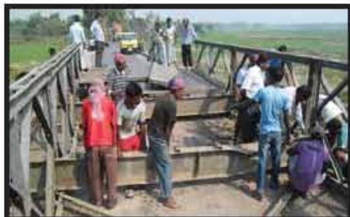
The workers are repairing the bridge.
