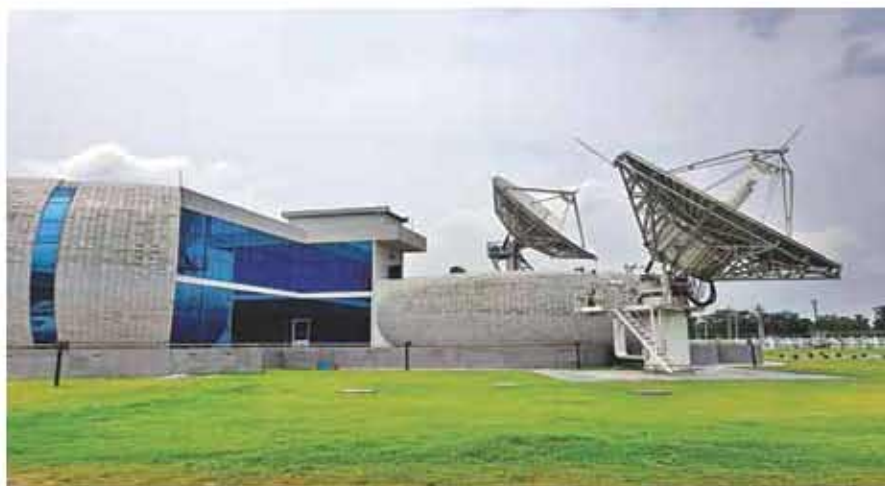
Ground Station of Bangabandhu-1 Satellite
